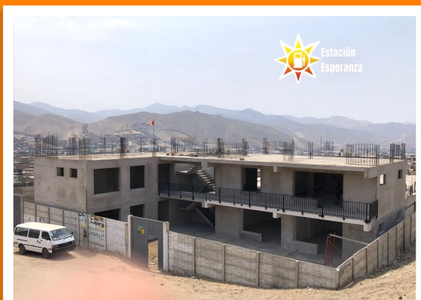
Progress in construction (kindergarten)
