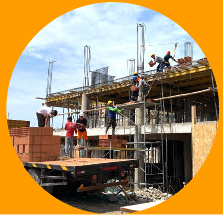
Progress in the construction
